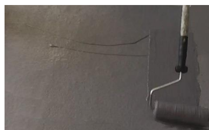
Second coat applied
