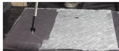
Wetting through the fibreglass CSM
