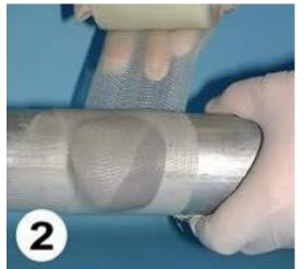
Apply the Eli-Wrap Bandage around the damaged area, extending up to 50mm (2") either side of the leak to ensure complete coverage. It is important that the bandage is applied quickly as curing begins once it is taken out of the water.
